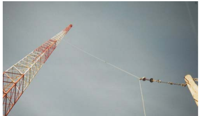
Figure 20a & b: Slant Wire Feed at KOAC
