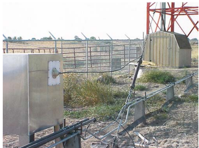
Figure 15: Slant Wire Feed and ACU Enclosure at KBKR
